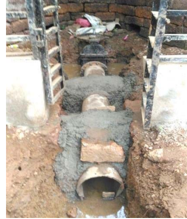
Figure 11: Restoration works of the Sluice Valve
